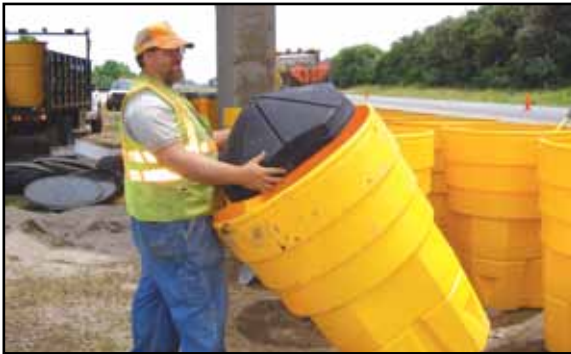
Figure A: Cone-shaped side always faces up.
